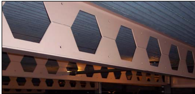
Castellated beams used in the adjacent Duquesne University Parking Garage
